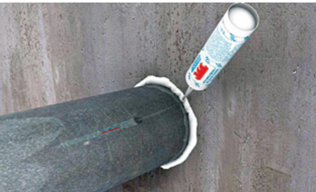
Fig 2 : Application of acrylic sealant at the joints for sealing purposes.
